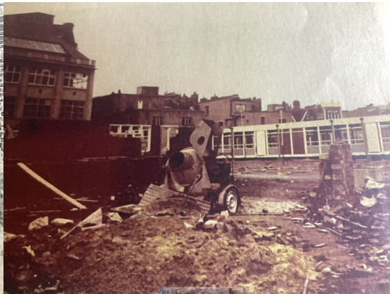
Old school being demolished, 1960s
